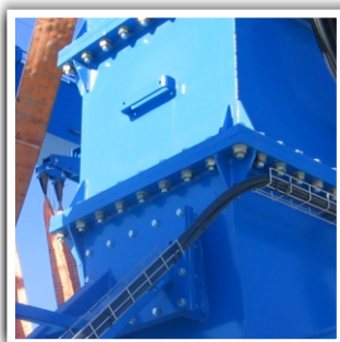
BOLTED STRUCTURE FOR EASY ASSEMBLY
